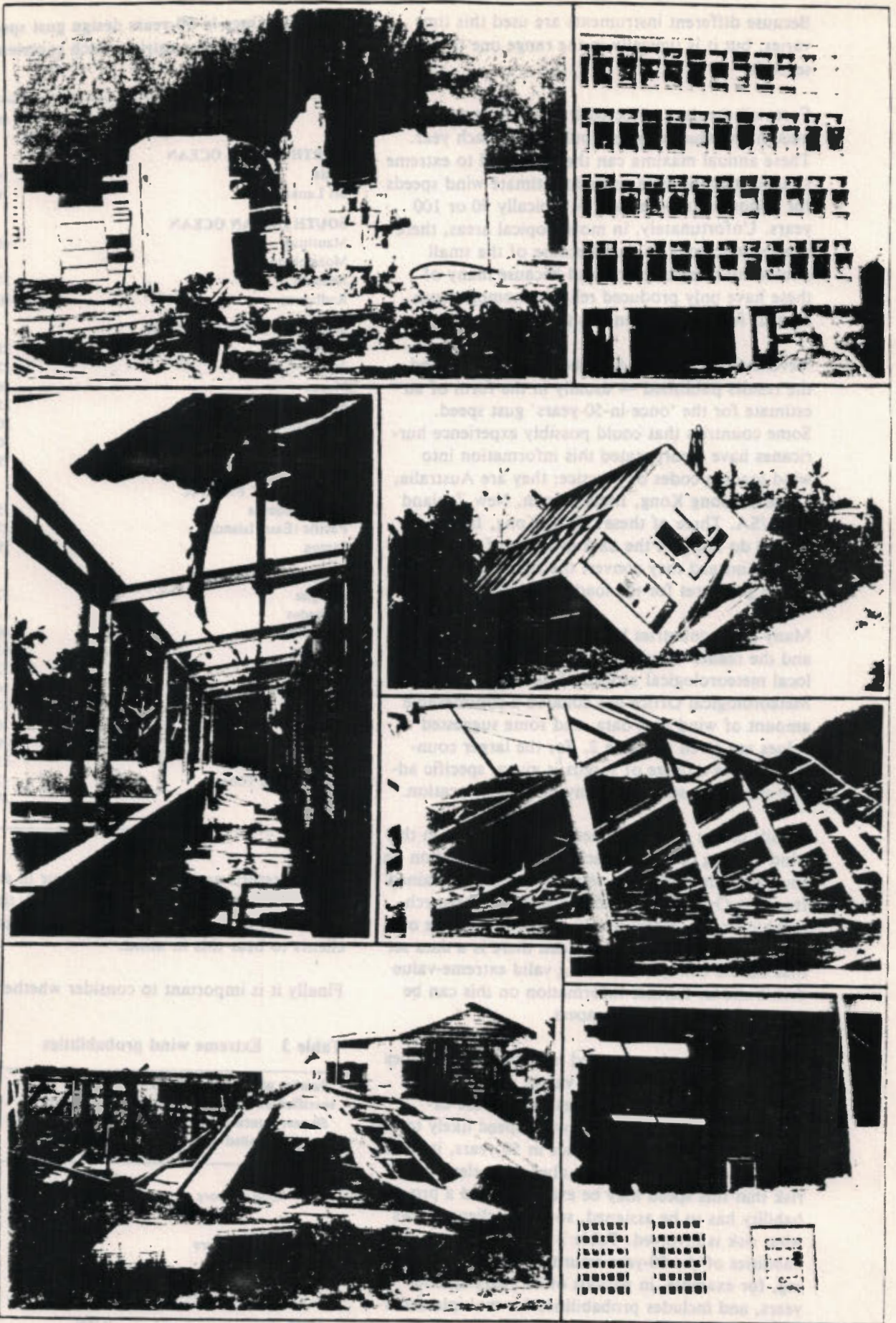
Figure 2 Examples of damage to buildings by hurricanes
